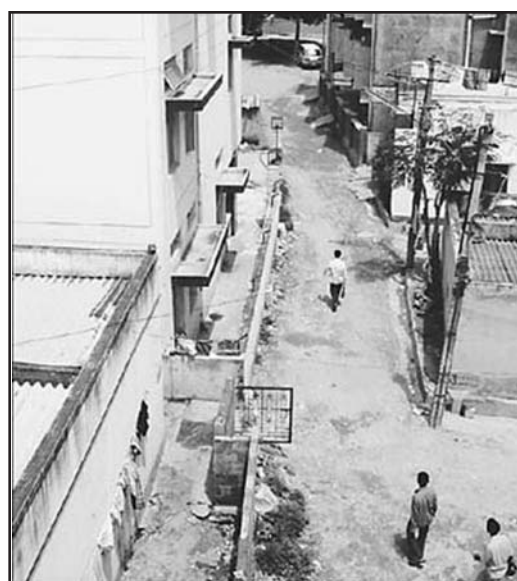
Undemolished illegal buildings Courtesy-Indian Express
